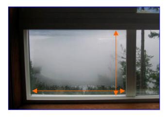
Here you see indicated by arrows vinyl touching glass to where vinyl is touching glass WxH– this is reffered to as 'DLO' or daylight opening. One inch is added to width and height to gain actual sealed unit size required. (or  $\frac{1}{2}$ " all way around more specifically)
