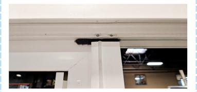
Install two #8 x 2 ½" screws through the frame tower through weather-strip slot at the sill at interlock end of the panel. See image for correct angle. Use caution to not over tighten which may strip screws.
