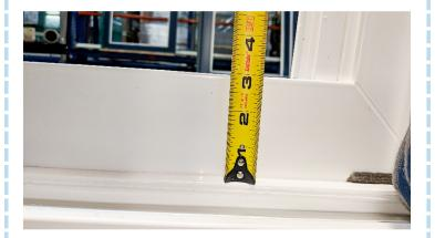
Install one #8 x 2  $\frac{1}{4}$ " screw into the jamb tower 3" up from sill, through the weather-strip slot.
